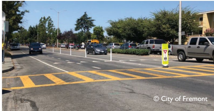
Figure 2. Graphic. Example of quick build crosswalk improvements. 1
